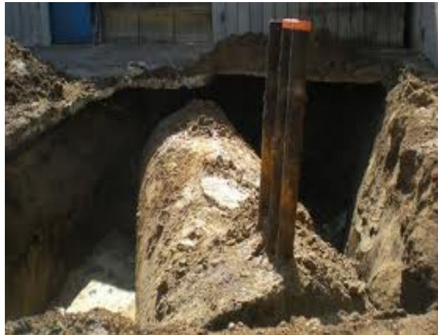
Figure 1 : Underground Storage Tank
